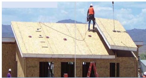
Figure 25: Insulfoam’s Structurally Insulated Panel
