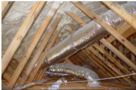
Figure 7: SPF Insulation Installation
