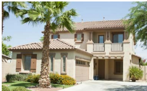
Figure 28: Finished Stucco
